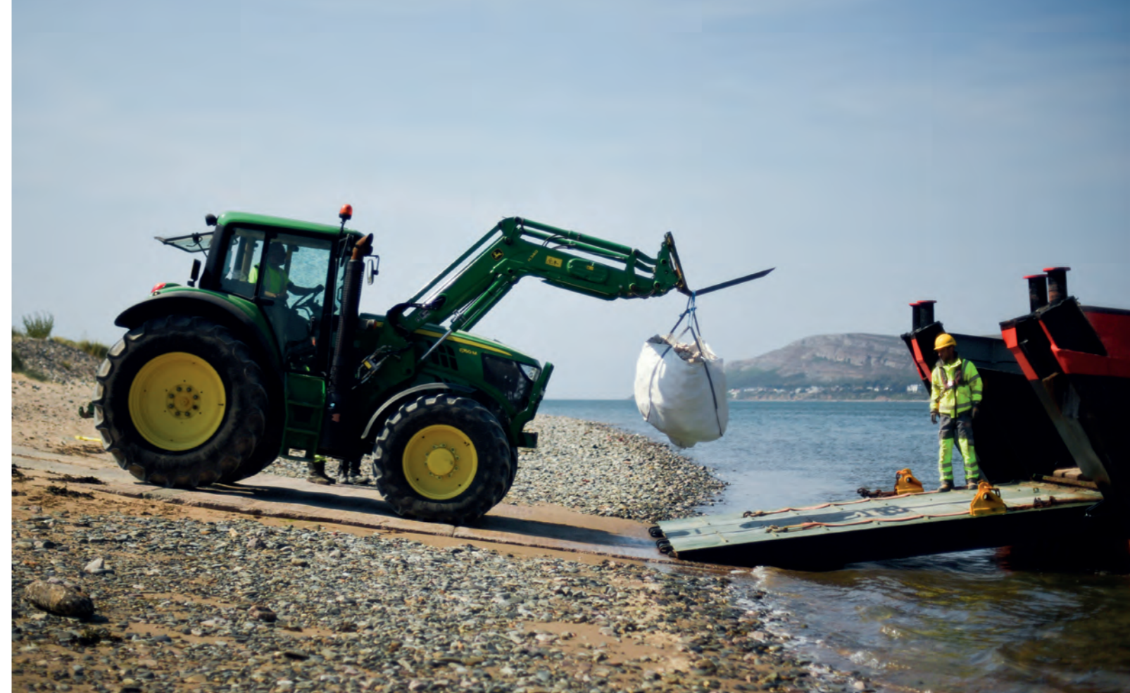
Main Photo: Loading of gravel cultch for the Conwy Bay reef. © Lucie Machin. Above: Limestone gravel cultch used to create the Conwy Bay reef. © Lucie Machin
